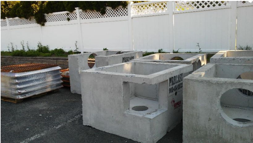
MS Site Work – storm drainage structures
