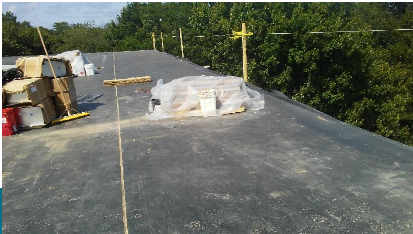
HS Addition – roof membrane in progress
