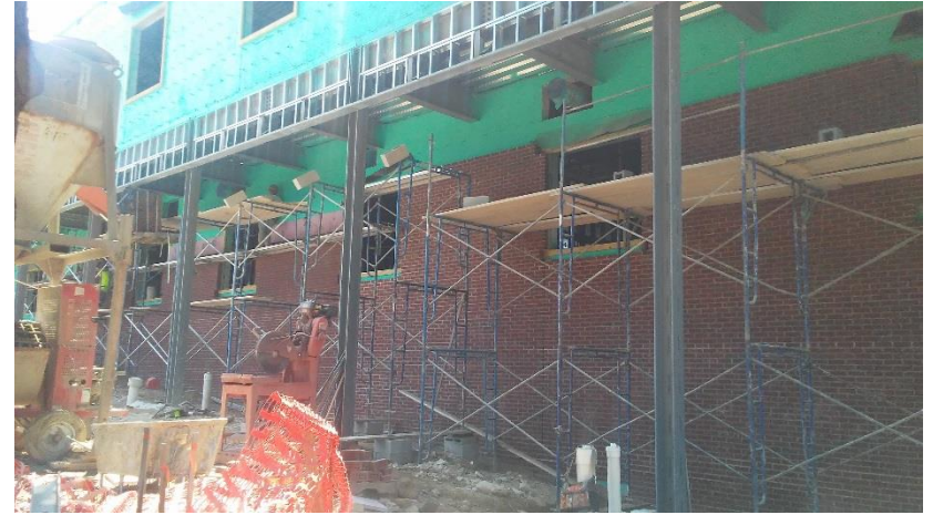
HS Addition – brick veneer and vapor barrier
