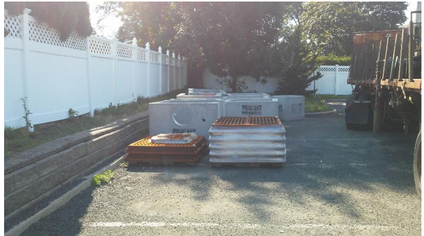
MS Site Work – storm drainage grates and structures
