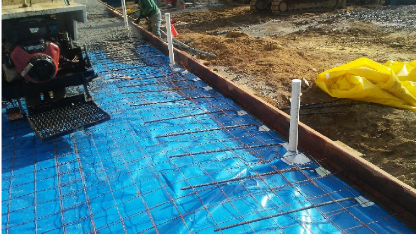
Preparation for first floor concrete slab
