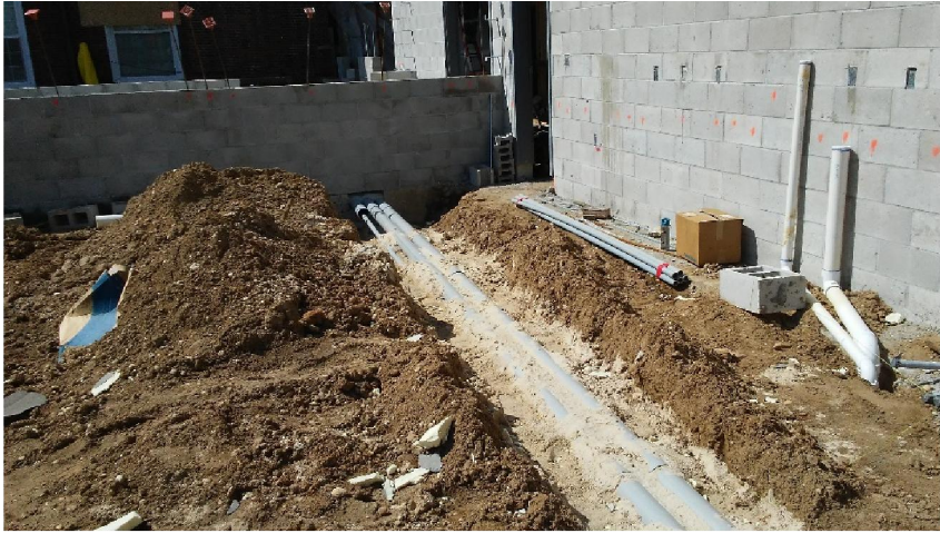
Electrical underslab rough-in
