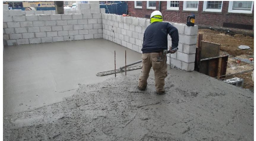
Stair tower floor slab in progress
