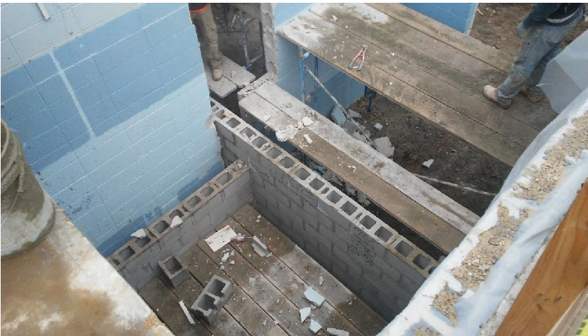
Elevator shaft block wall in progress
