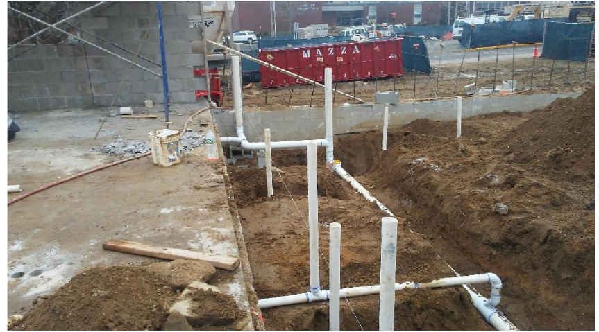
Underslab sanitary plumbing rough-in
