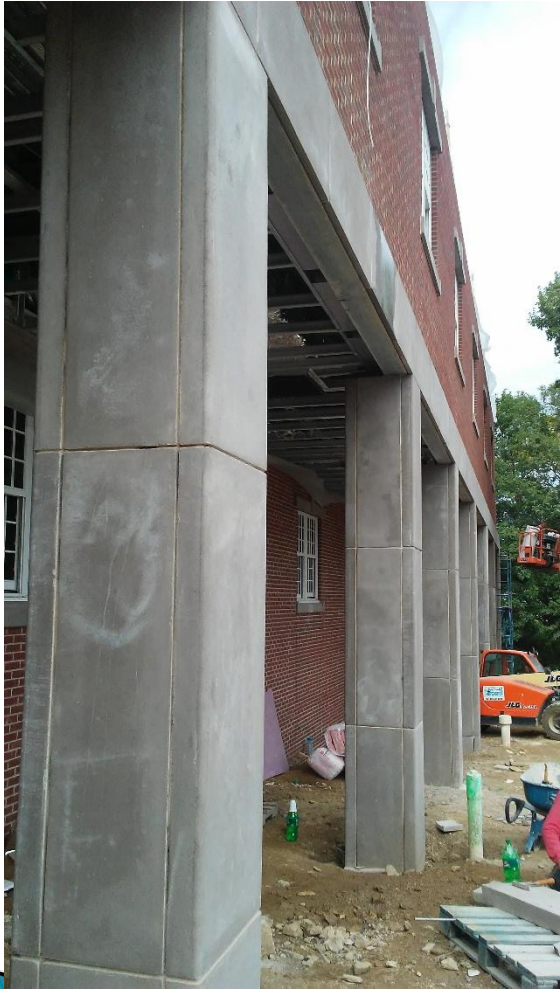
HS Addition – cast stone column covers in progress
