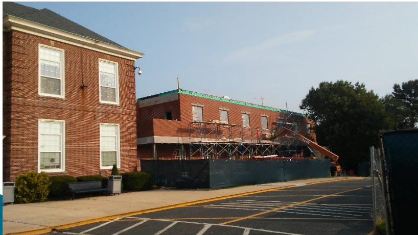
HS Addition – Masonry veneer near completion
