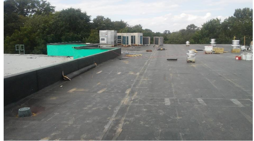
HS – EPDM roof on building addition
