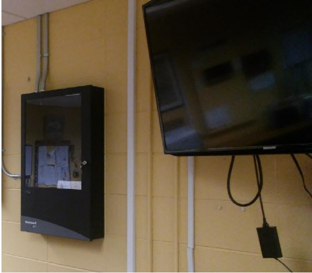
ES Fire Alarm Control Panel
